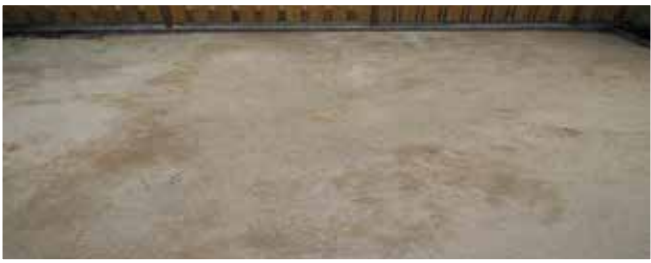
Step 1 – Apply Foundation For Artificial Grass
